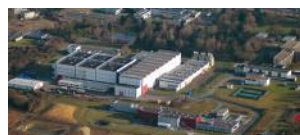
GANIL-SPRAL2 facility in Caen, Normandy
